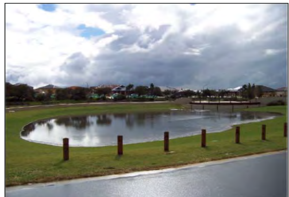
(Top left) Dry basin landscaped swale within multiple use function restricted use public open space (Top right) Landscaped dry basin in POS after storm event
