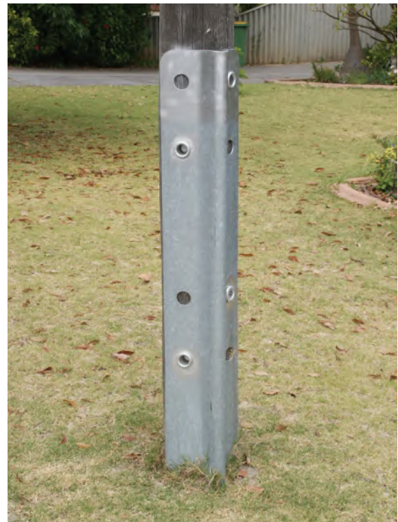
Figure 5 – Typical reinforcement of timber poles with steel supports
