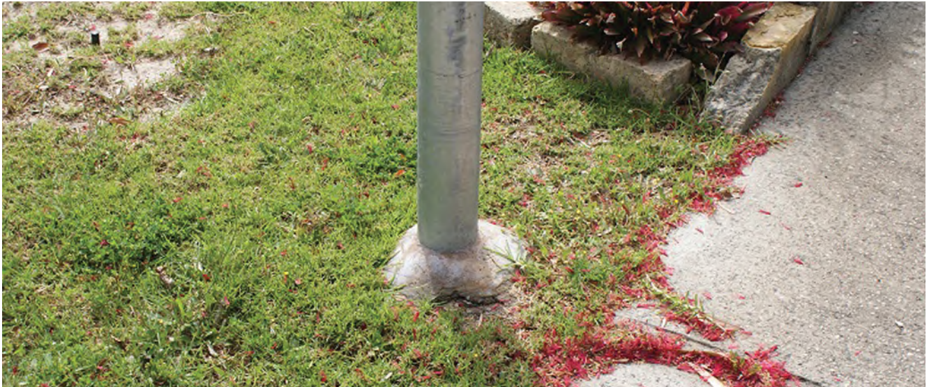
Figure 7 - Correct installation of steel pole with concrete footing finished above ground
