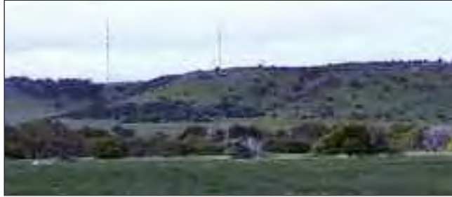
Figure 12: Existing telecommunication towers on the range are relatively inconspicuous.
