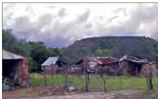
Figure 7: Historic buildings indicate previous settlement patterns on the range's foot slopes.
