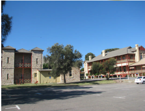
Bill Sewell Complex
