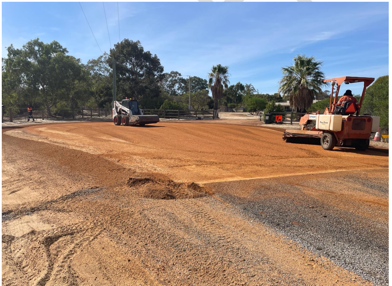
Example of Resurfacing Works – Ridgeway Close – Moresby 2024
