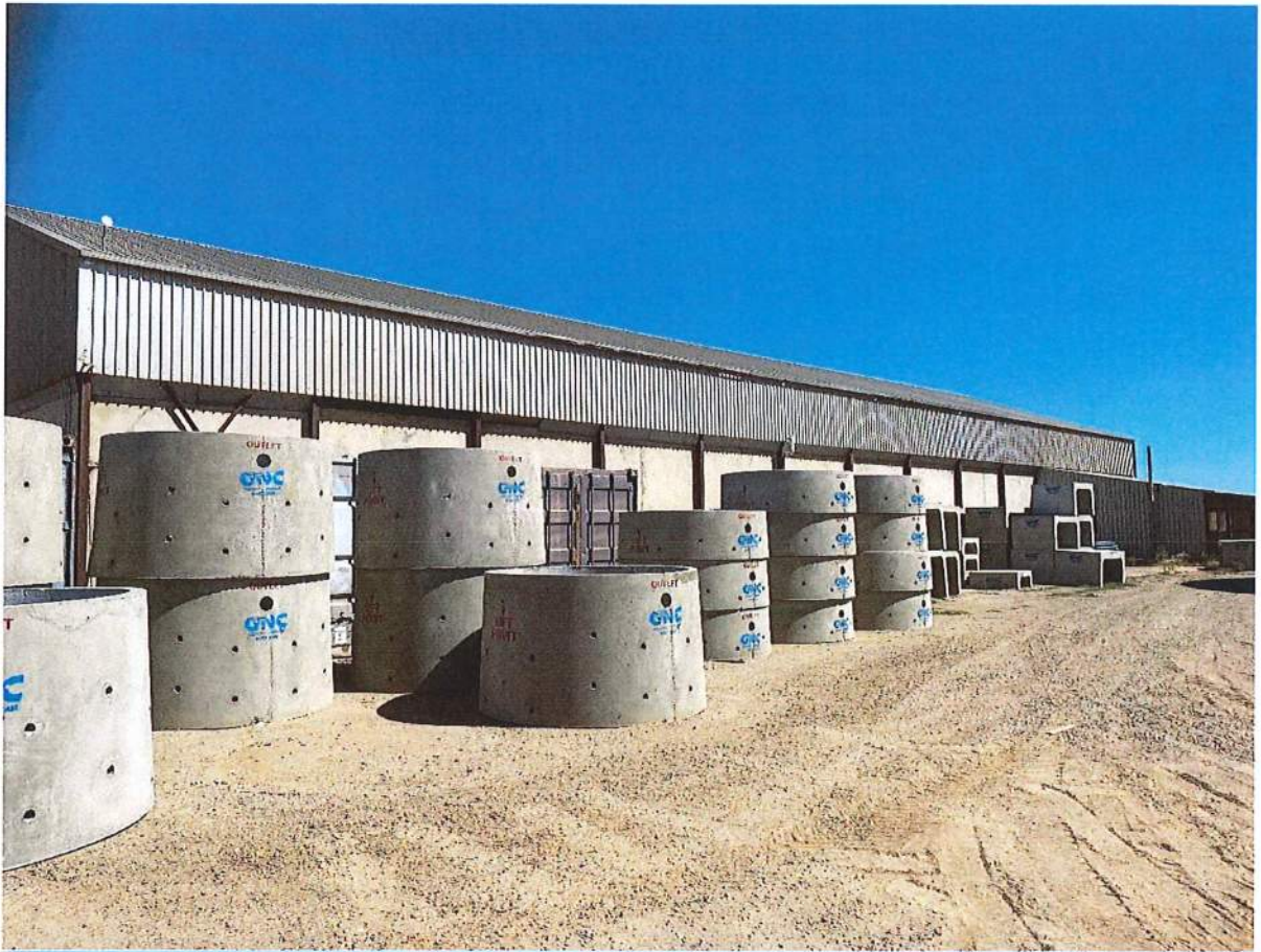
Photos of site inspection conducted at 34317 Brand Highway South Greenough (Martins Mill) Fiona McAuliffe & Andy Gaze Tuesday 16 April 2024 (Steve Easton Present)
