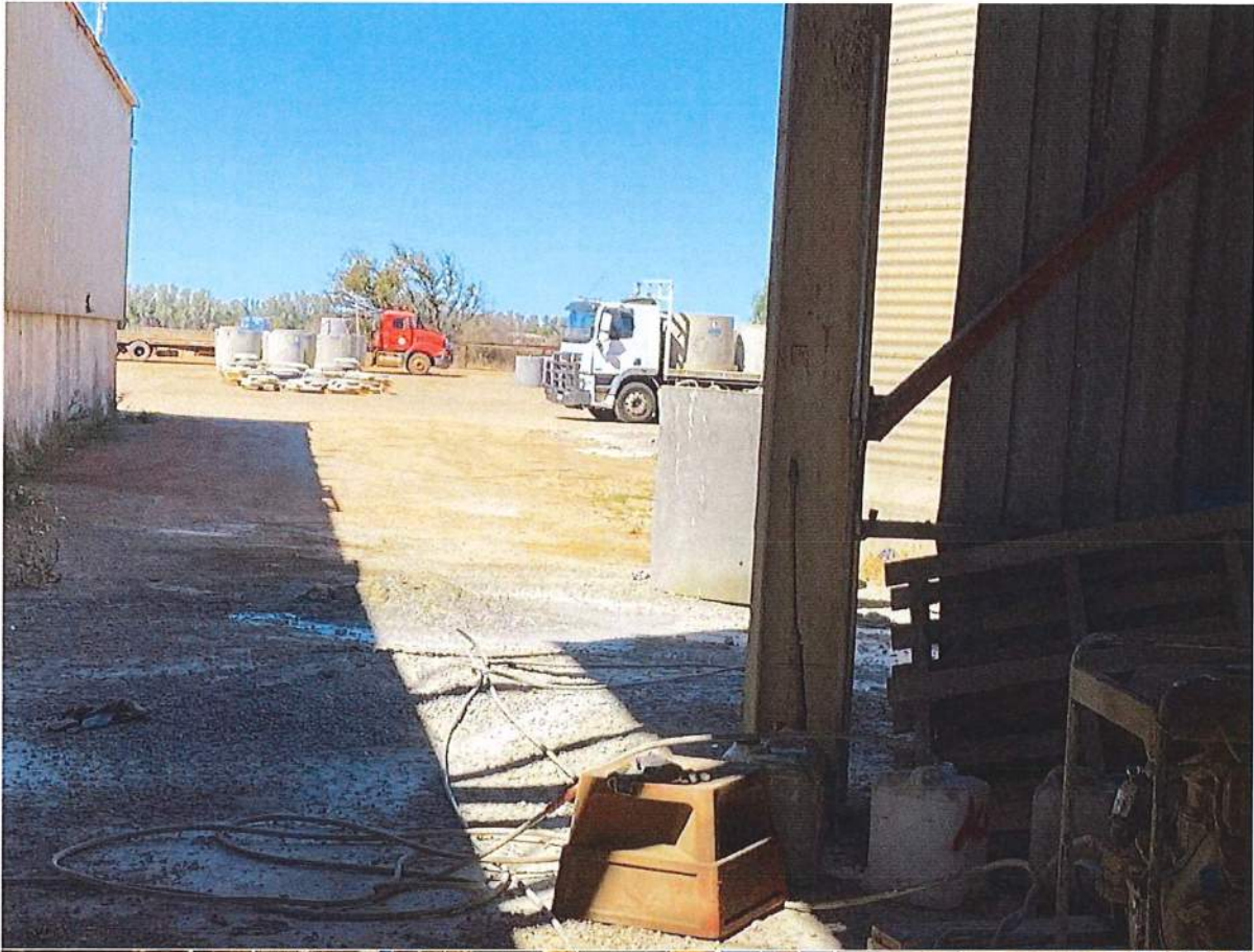
Photos of site inspection conducted at 34317 Brand Highway South Greenough (Martins Mill) Fiona McAuliffe & Andy Gaze Tuesday 16 April 2024 (Steve Easton Present)
