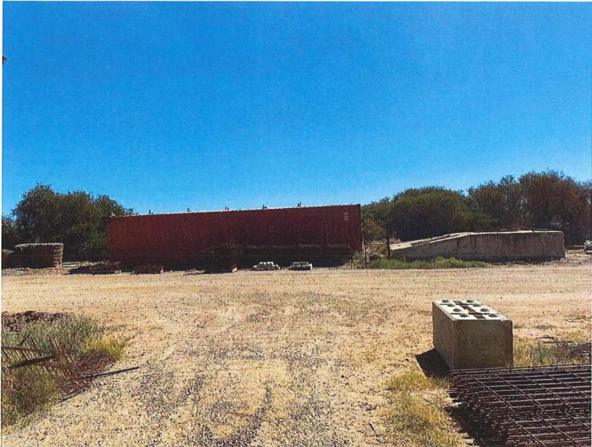
Photos of site inspection conducted at 34317 Brand Highway South Greenough (Martins Mill) Fiona McAuliffe & Andy Gaze Tuesday 16 April 2024 (Steve Easton Present)
