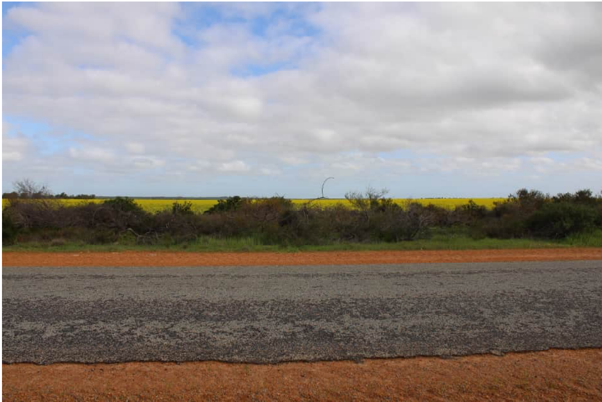
Plate 6: Site 5 – Middle of Project Area (Walkaway-Nangetty Rd)
