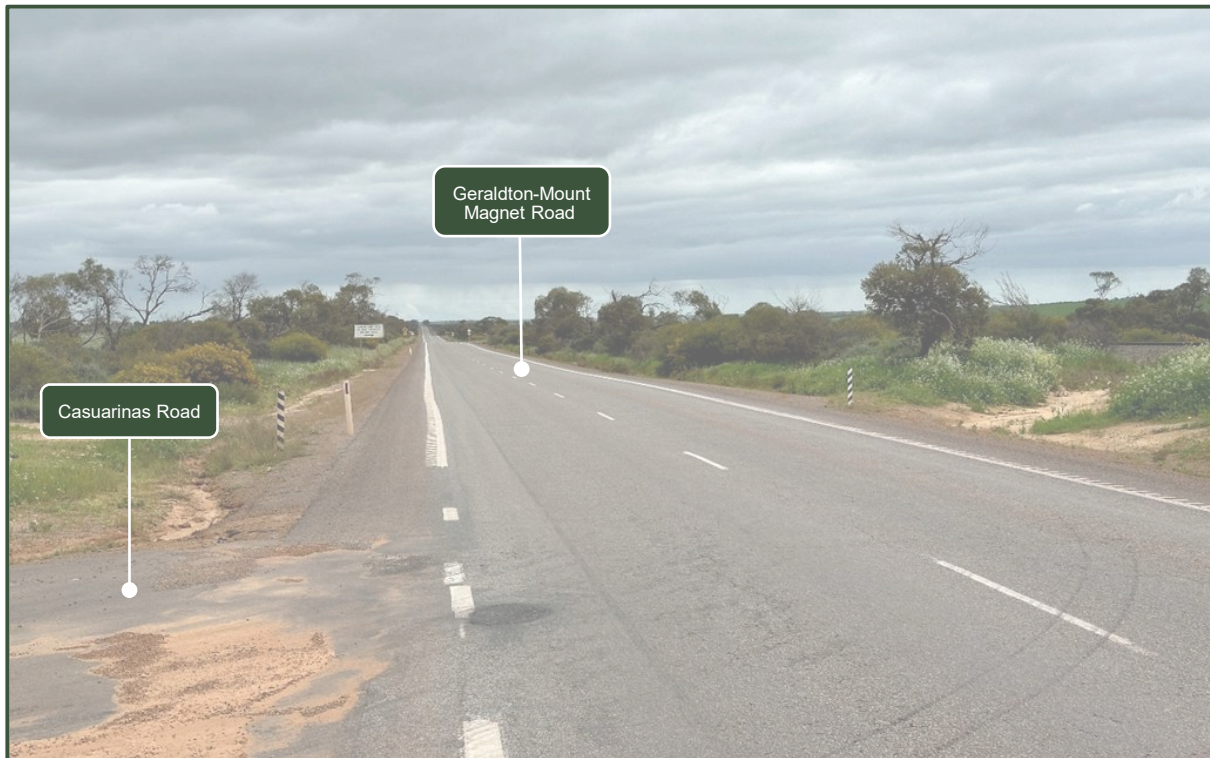
Figure 4 Geraldton-Mount Magnet Road (Facing West – 20/08/2024)
