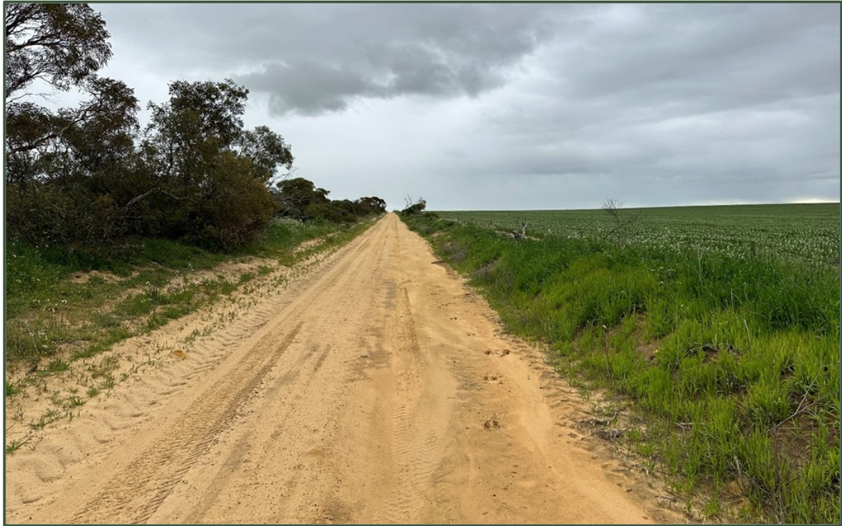
Figure 8 Edwards Road (Facing West – 20/08/2024)
