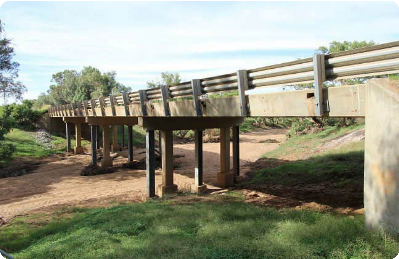
Above: Nangetty-Walkaway Rd Bridge over Greenough River, Walkaway. (Source: City of Greater Geraldton)
