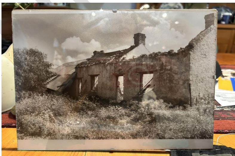
Image of the remnants of the cottage prior to restoration and additions. Courtesy Richard Jones.
