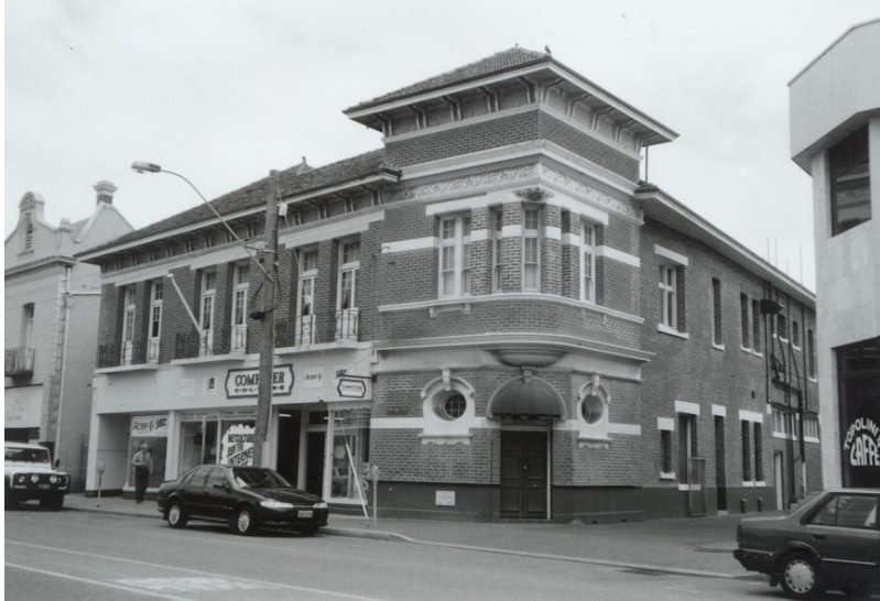
Photo Description: 30/10/1996 Suba, Callow & Grundy Balconies removed.
