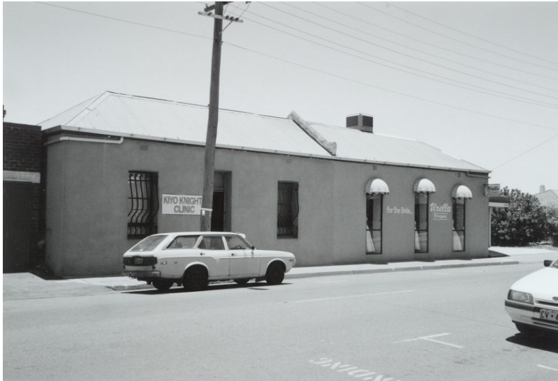
Photo Description: 8/12/1996 Suba & Grundy View from Lester Avenue.
